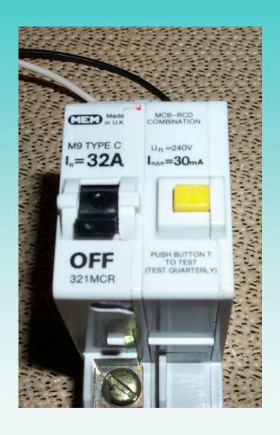
single device provides protection against both overload, short circuit and earth fault currents
