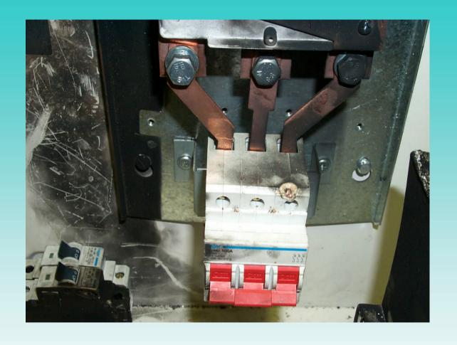
Result of electrician fitting circuit breaker to live board
