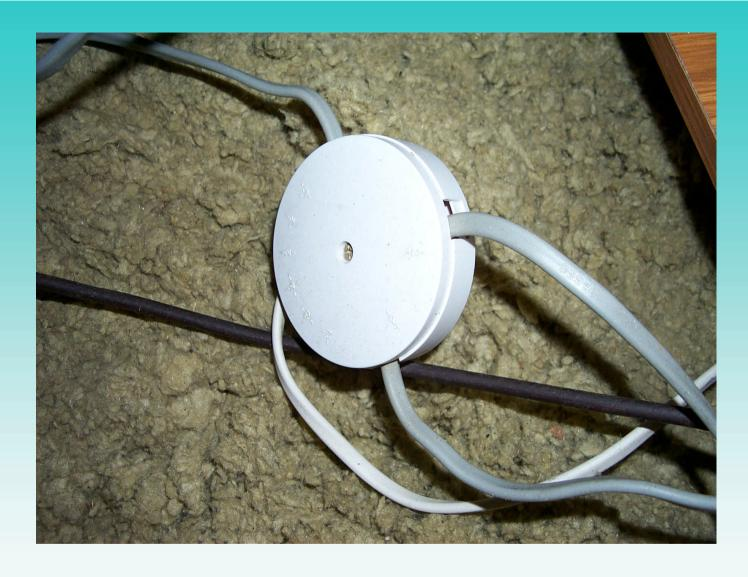
circuit connections may be dislodged by movement of the joint-box.
