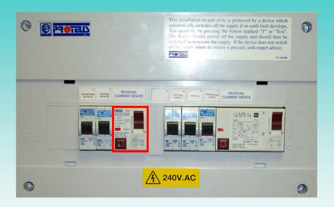
Second r.c.d. has greater sensitivity and is used to protect socket outlet circuits
