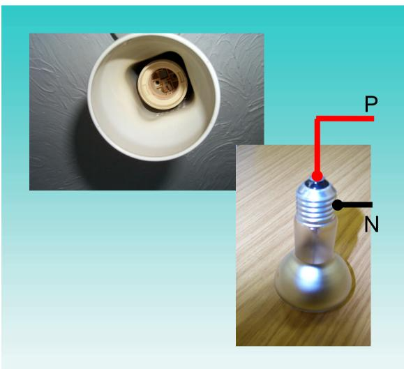
Centre contact must always be connected to the phase conductor of the supply
