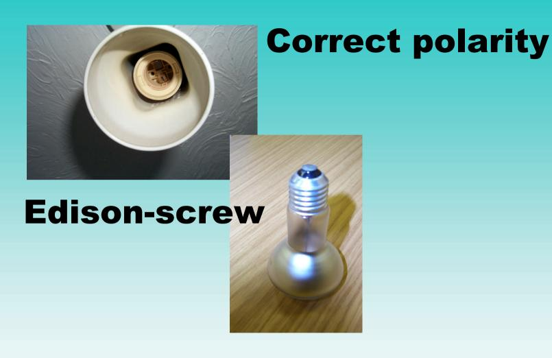
Correct polarity of Edison-type screw fittings essential if shock is to be avoided
