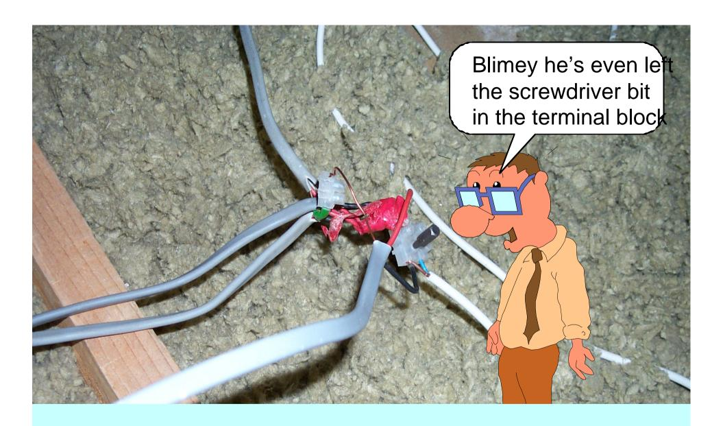
potential fire/shock risk due to mechanical damage or loose connections
