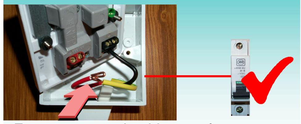
Excess current should cause fuse or circuit breaker to operate
