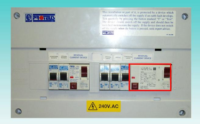
Least sensitive of the two devices and protects circuits feeding fixed equipment.
