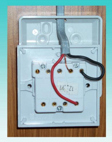
When converting one-way to two-way lighting the earth wire used as live conductor
