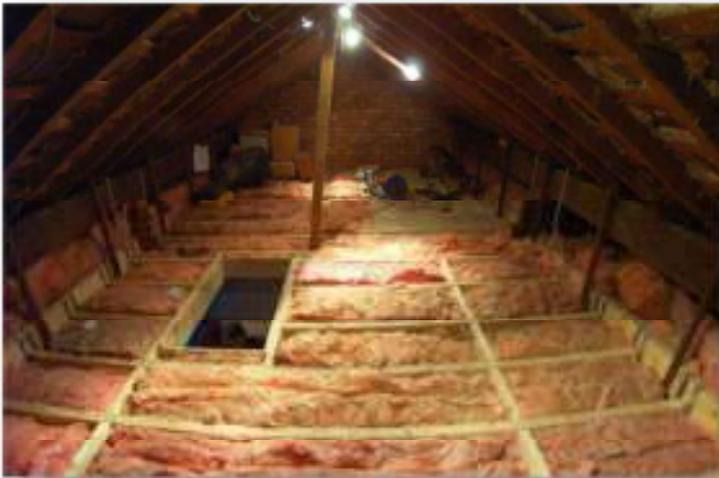
**Thermal Insulation** – If a cable, through any part of its run, passes completely through thermal insulation this can greatly impede its ability to dissipate heat generated through current flow. Therefore regulation 523.7 identifies corrections to be made for this situation. The symbol for correction factor for thermal insulation is **Ci**.
